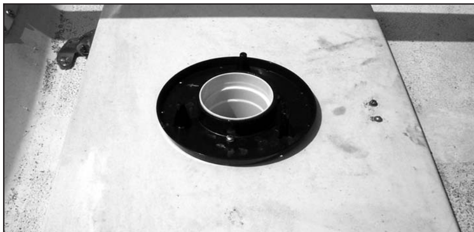
Pictured above is the vent base fastened in place.
