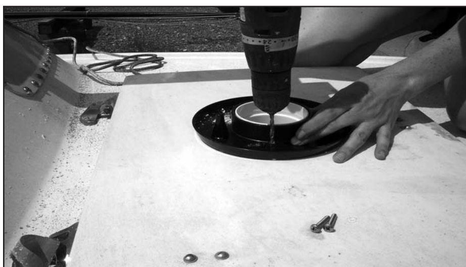
One part of this process includes drilling mounting holes.
